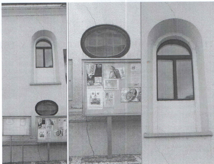
Figure 1: The splits and tears on the church
